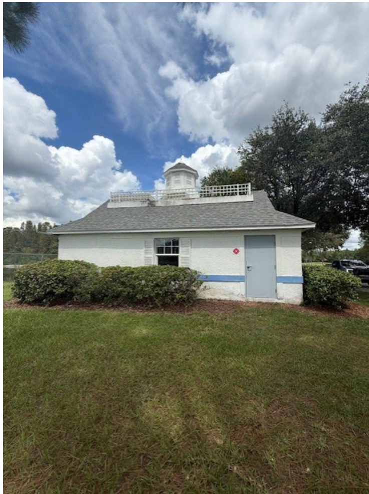
Pump House Next To Driving Range
